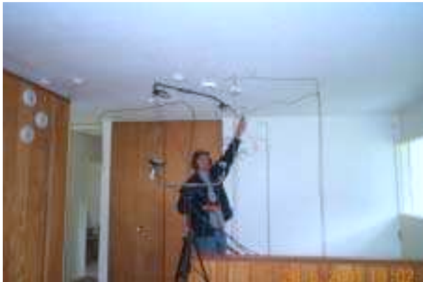
Installing different technology smoke detectors in house.
